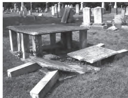
Time and erosion can lead to collapse
