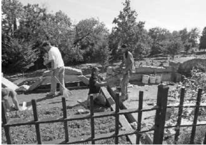
Installation of green roof in September 2014.
