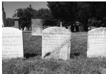
McCaffrey tablet after repair.
