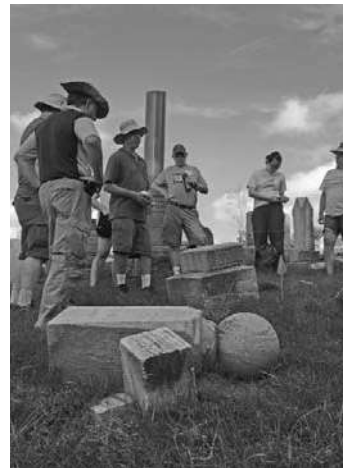
McDonald monument before repair.
