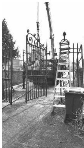
Removal of 1856 gate.
