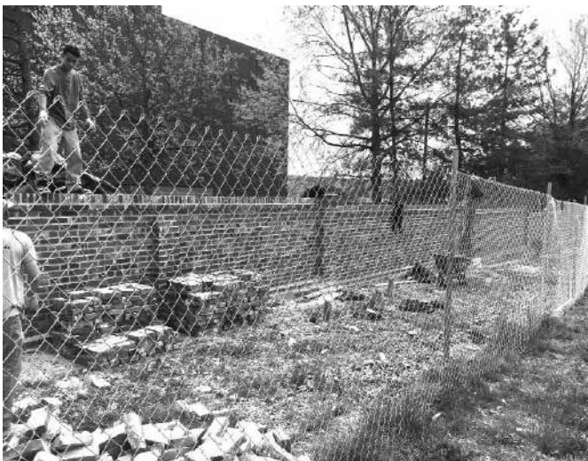
Finishing construction of new wall.
