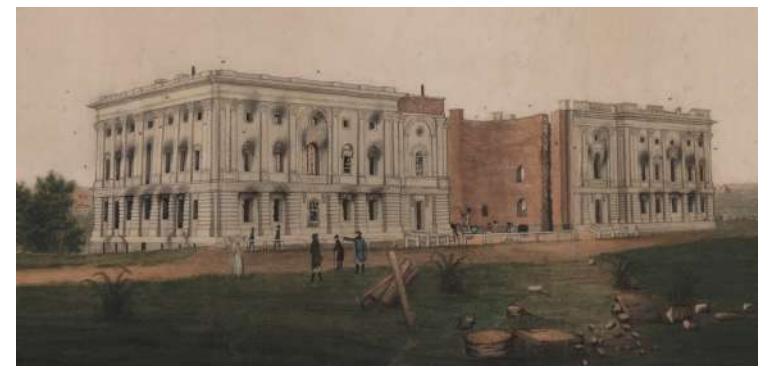
George Munger's drawing of the U.S. Capitol after burning by the British, including fire damage to the Senate and House wings, damaged colonnade in the House of Representatives shored up with firewood to prevent collapse, and the shell of the rotunda with the façade and roof missing.
